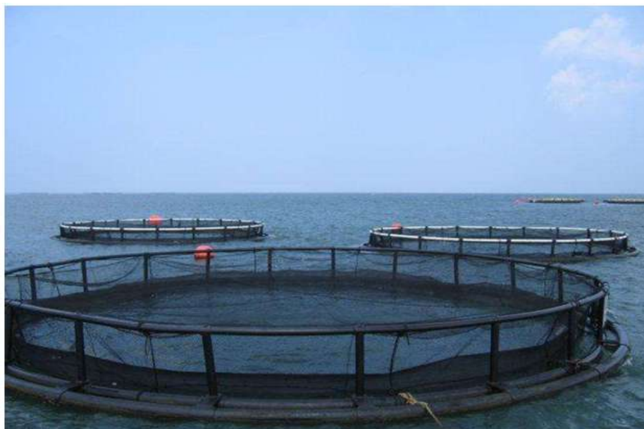
Figure1.2 Lifting deep sea cage
